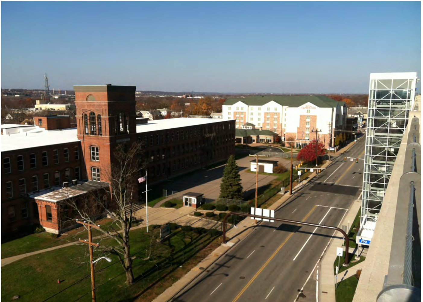
View looking northwest from the top of the Interlink garage. Elizabeth Mill/Leviton in the foreground, Hilton Garden Inn towards the back.
