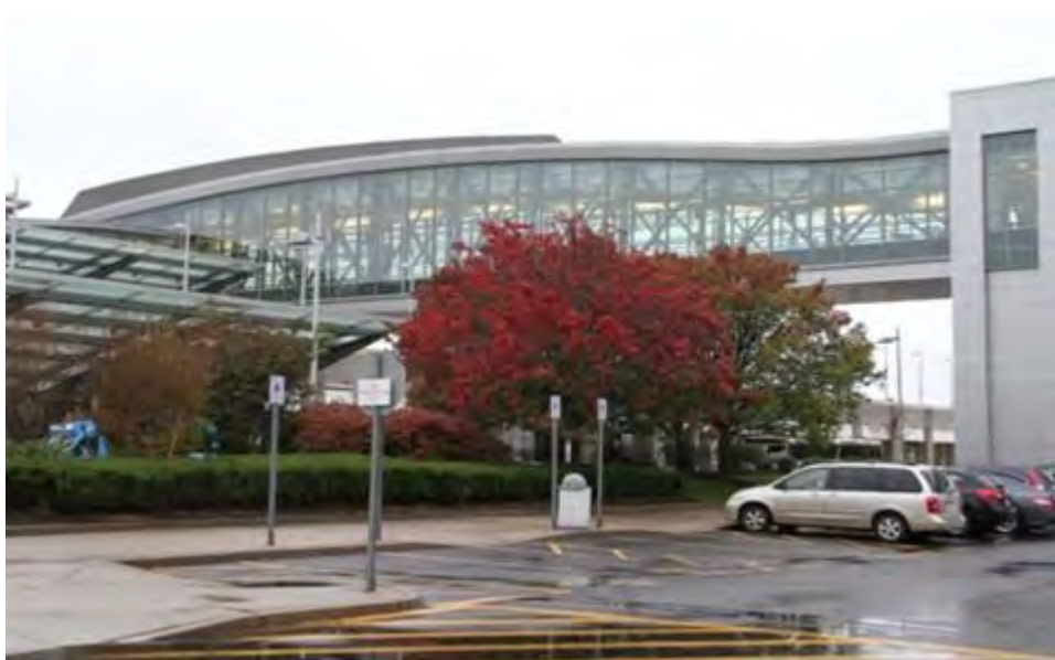
Photo courtesy of Chuck Aube, Rhode Island Department of Transportation
