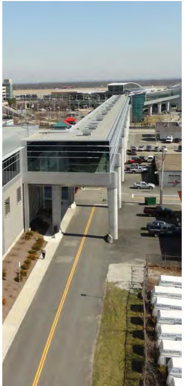
The Warwick Interlink. (photo source: www.siteselection.com )
